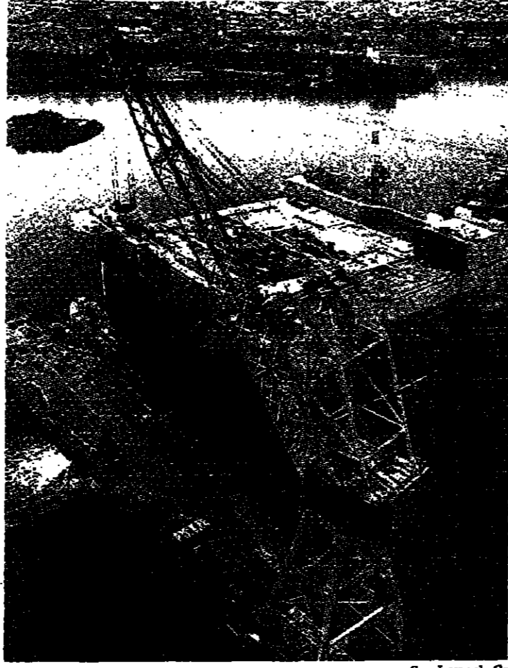
Boeing's mobile satellite launch site - a converted oil drilling platform
